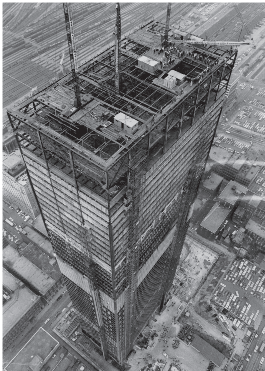
The Toronto-Dominion Centre under construction, 1966. Toronto Star, Boris Spremo / Contributor
